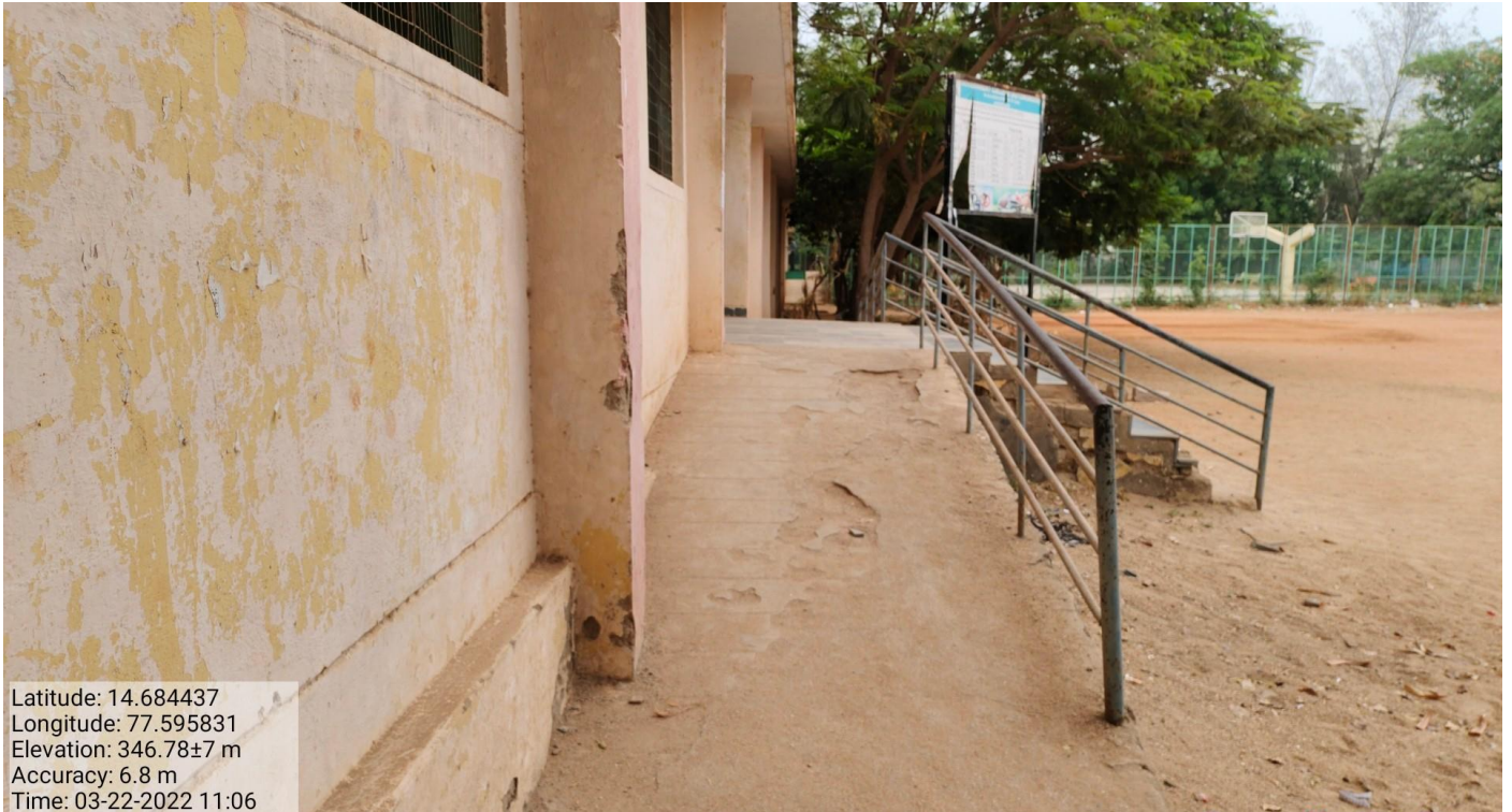
Ramp provided at Commerce Department
