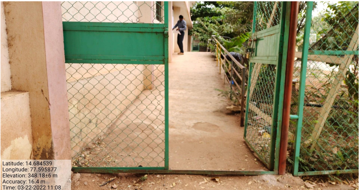
Ramp provided at Physical Education Department
