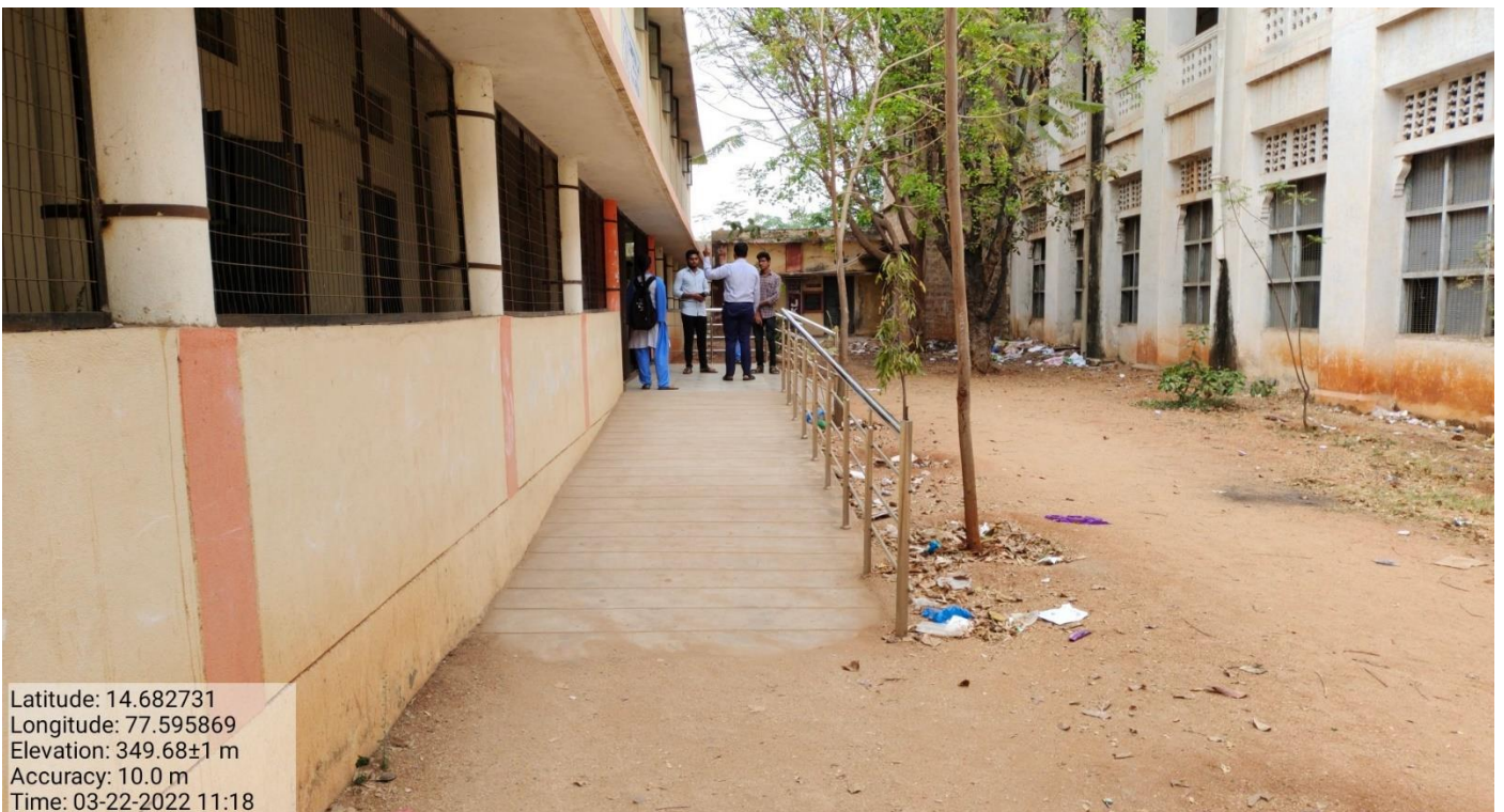
Ramp provided at RUSA building
