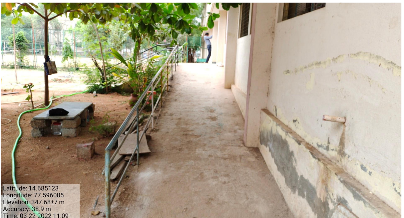
Ramp provided at Physical Education Department
